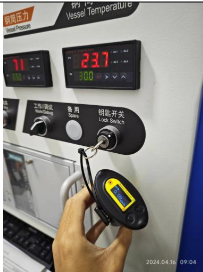
1#加速器主控柜上钥匙开关
