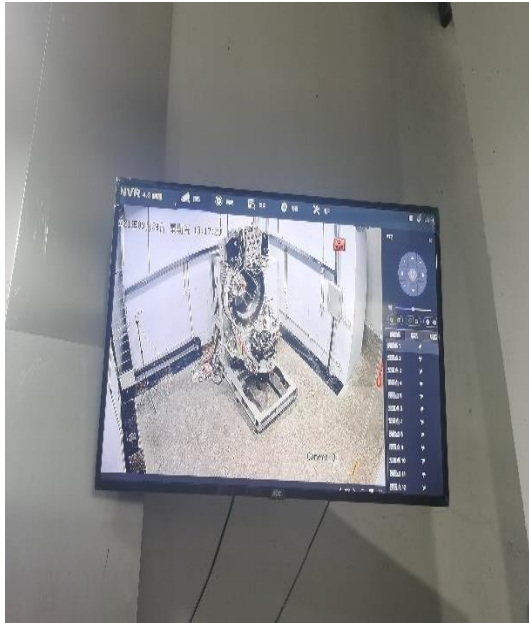
监控系统显示屏
